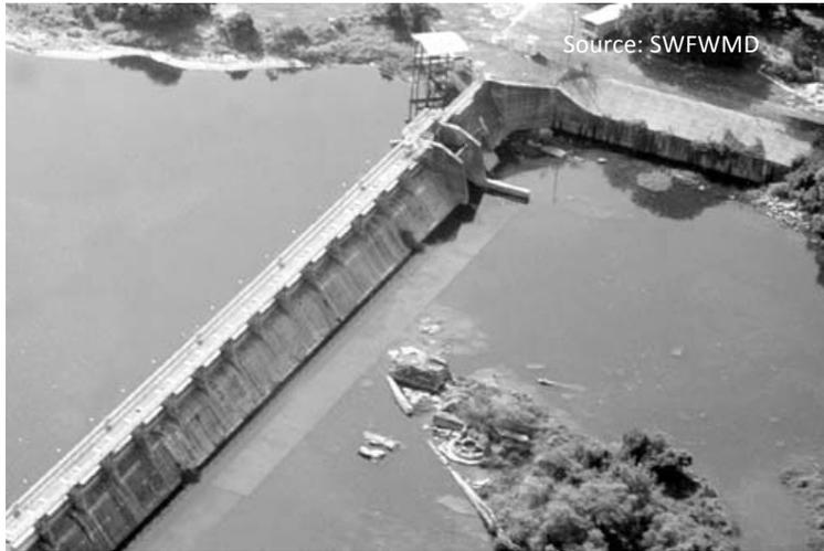
South of 40<sup>th</sup> street, the river gets wider and deeper. The reason is the City of Tampa Water Department’s dam. This dam interrupts the flow of water and creates a reservoir from which the city draws much of its drinking water supply. During drought years there isn’t any flow of water over the dam. The Southwest Florida Water Management District has a plan to restore a minimal flow of water at the dam into the lower Hillsborough River.
